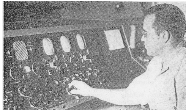
Figure 7. Cathode ray oscilloscopes used for monitoring carrier of each transmitter. These are mounted in the control desk.
