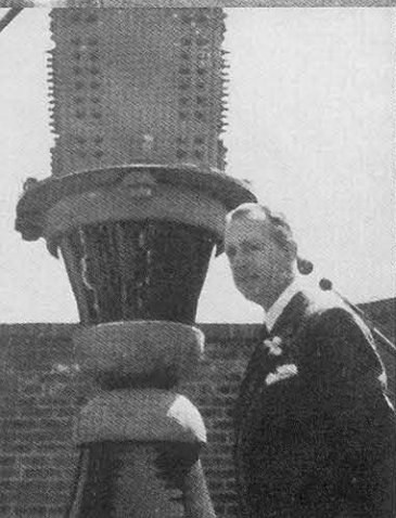
Powel Crosley, Jr., photographed at the base of the 831-ft. antenna of 500,000-watt WLW. The two cup shaped porcelain insulators, with walls less than two inches thick, support a stress load of more than 900,000 pounds.
